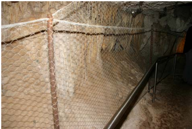
A small section of old wire netting in Mulwaree Cave retained for historical interpretation. Note the new stainless steel railing in front.
