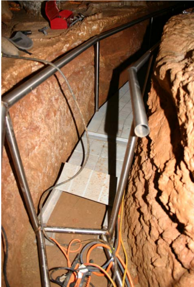
Track work in progress – Paddy Fields Section, Wollondilly Cave
