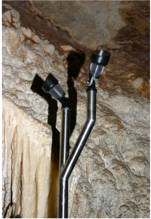
New light fittings on stainless steel poles – Star Chamber, Wollondilly Cave
